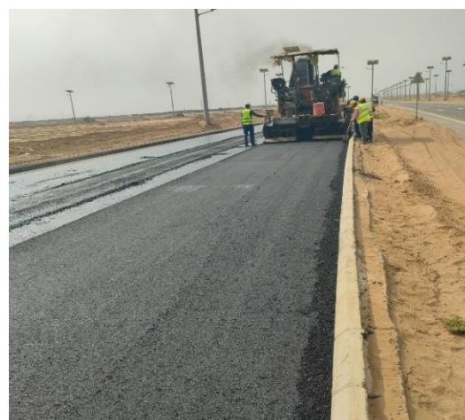
Applying the wearing course at road 7, and complete service road all along.
