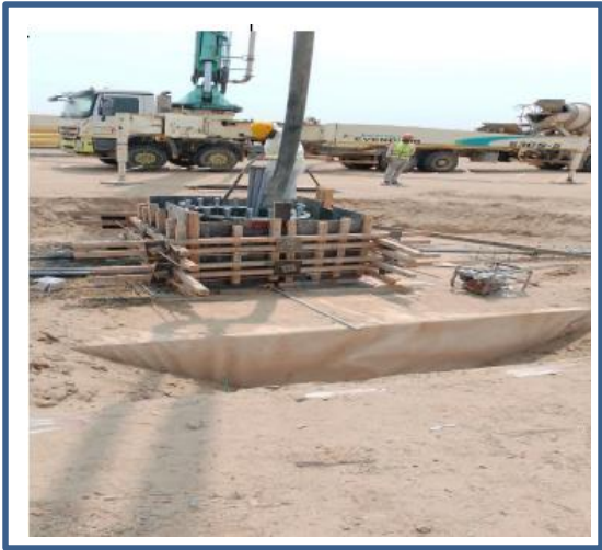
Concrete Pouring of High Mast Poles
