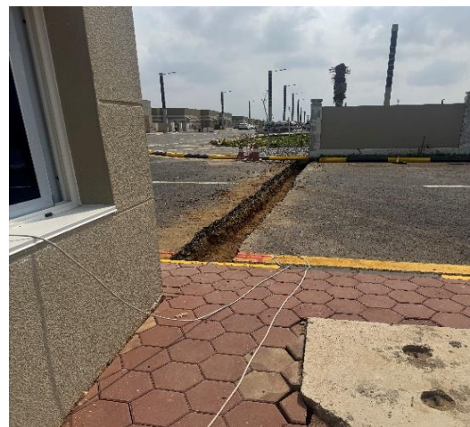
Main gate ground beam work
