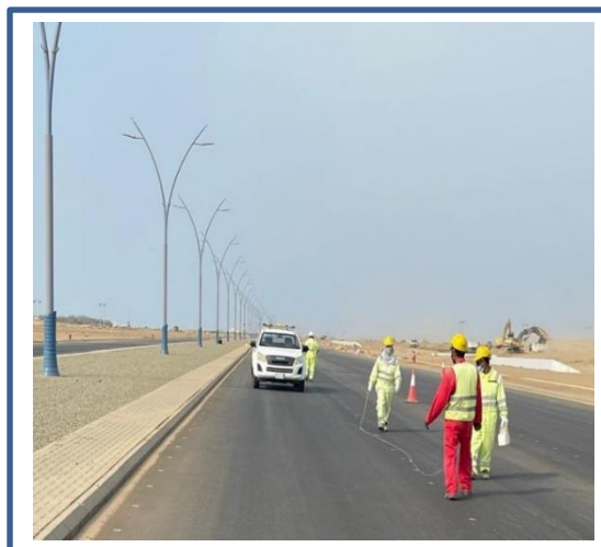
Measurement and Outline for the Road Marking
