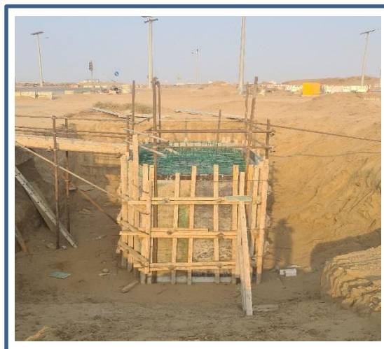
Ready for concrete pouring of top slab and walls for telecom MH # 21 and 25 between Road-7 & Road-7a Phase-2
