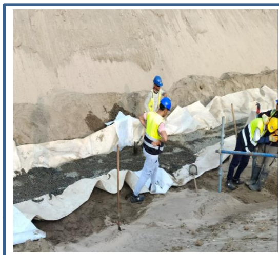
Installation of Geotextile around SWW pipeline
