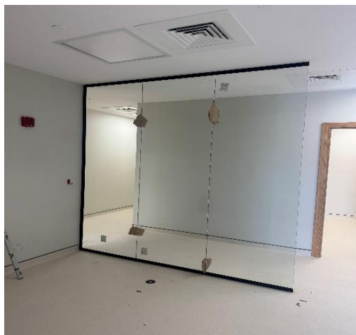
Installation of glass partition works in Clinic Building
