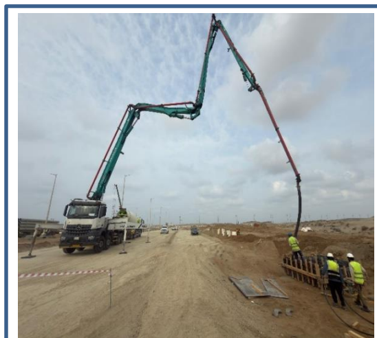
Pouring of Concrete for Top Slab o Catch Basins in Zone-2
