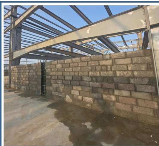
Masonry work at block 4
