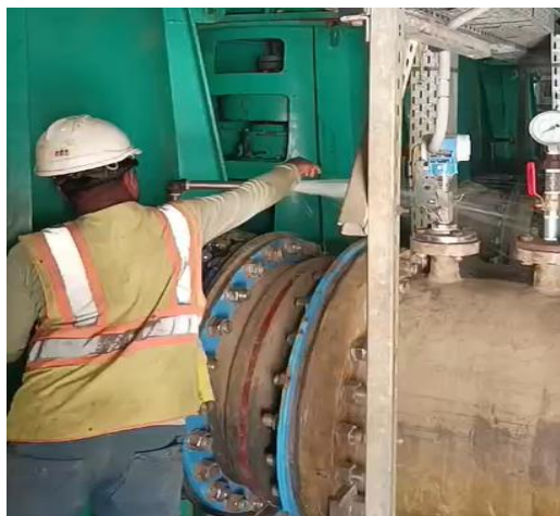
Testing of Pump #04 after completing repair
