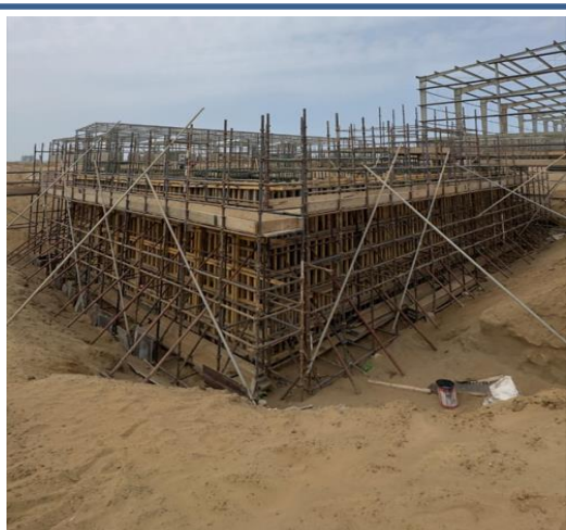
Water tank shuttering and concrete pouring
