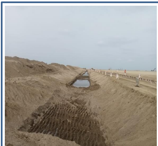
Excavation for sewer line
