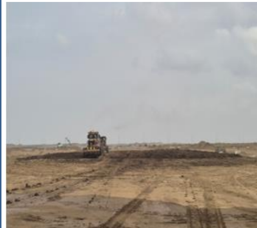
MJR-04 grading of backfilling soil material
