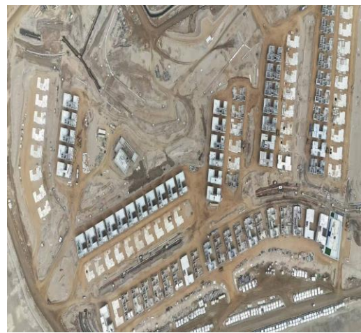
Overall view of project site construction
