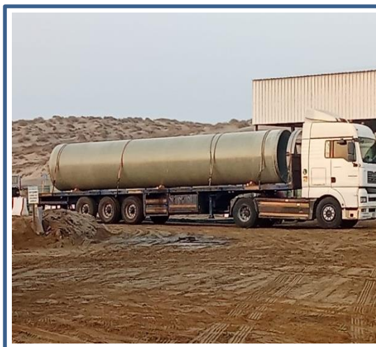
Delivery of SWW pipes to site
