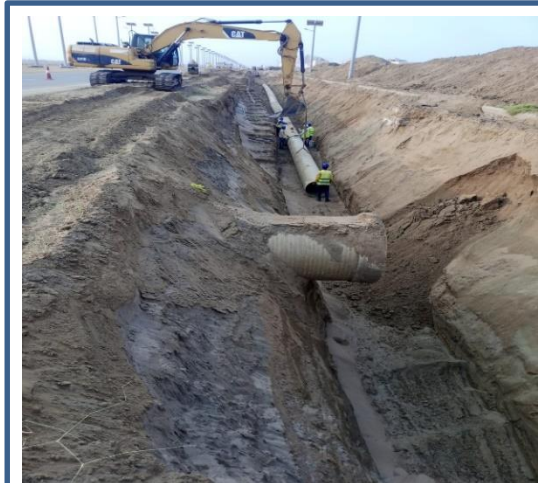
GRP Pipeline Installation at Road-01
