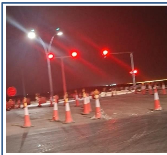
Functional Test of the Traffic Signal System at Road 5 and Road 8 Intersection
