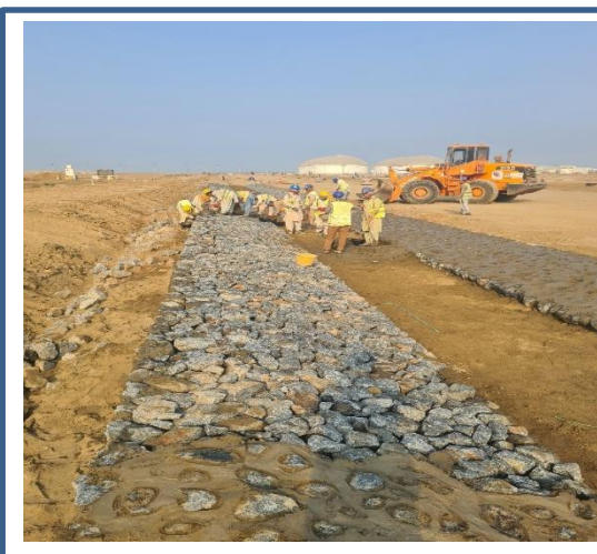
Grouting of stone rip-rap (swale) onward to Road-1, south side of carriageway
