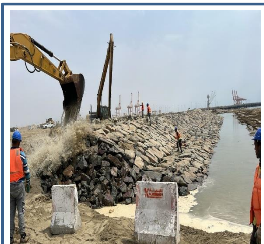
Revetment construction
