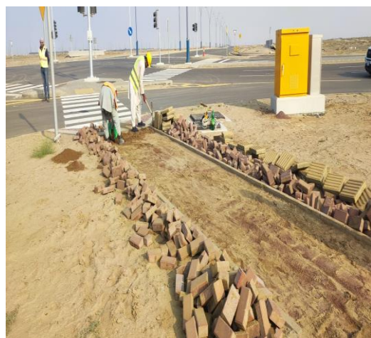
Hardscape closeout works in walkway areas, intersection road 01, 03 and 05 (Interlock, tactile, curbstones)
