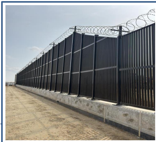
SS Boundary / decorative fence installation completed
