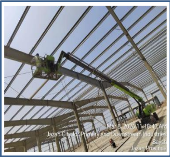
Main warehouse Structural Steel Painting
