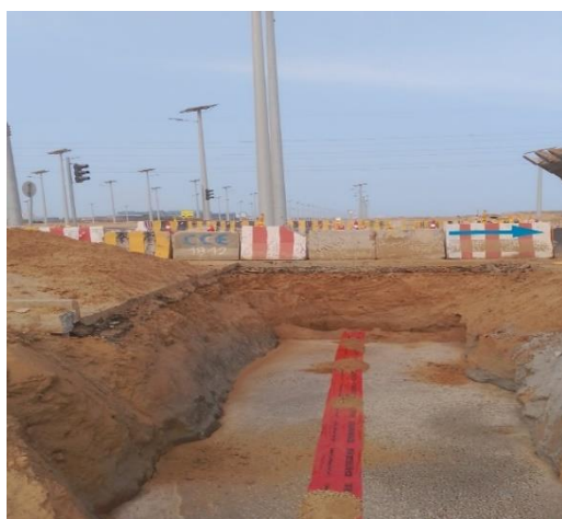
Completing pipe encasement after pipe installation & testing and backfilling.
