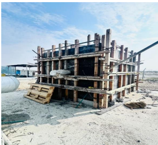
Formwork for outer walls for Concrete Chambers ongoing at Laydown Area.
