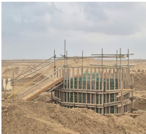
Formwork and steel fixed for telecom manhole
