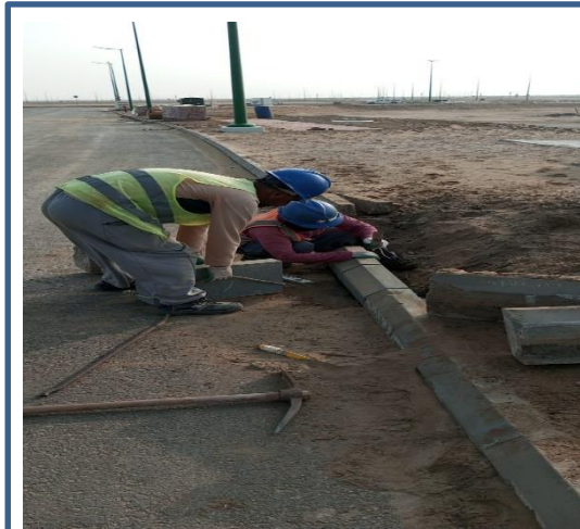
Repaired damaged Curbstone Road HR1-1
